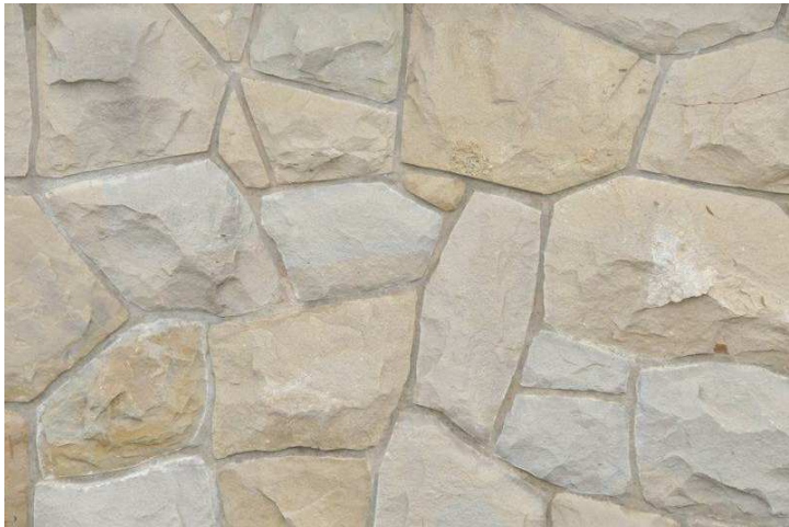
Code: EW5 Material: Existing Loose Sandstone Retaining Wall Disassembled and Rebuilt with Mortar Location: To Form Lower Part of Plinth
